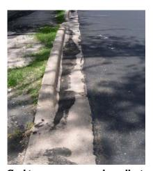
Coal tar overspray powder collecting at edge of lot. Breaks in curb allow easy access to streams.
